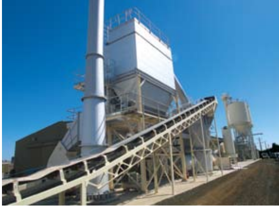
✓ RAPIDFLOW CALCINATION PLANT, KILMORE VICTORIA.
