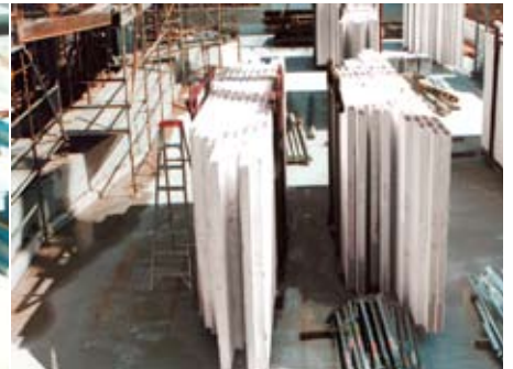
▾ WALLS PLACED AND PROPPED BEFORE ▾ PLACEMENT OF FLOOR FORMWORK
